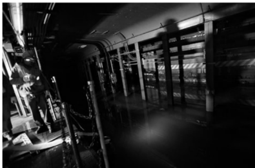
Workers pumped water out of the South Ferry subway station at the tip of Manhattan, which was filled with water up to the ceiling after Hurricane Sandy struck. Go to related articles Hiroko Masuoka/The New York Times
